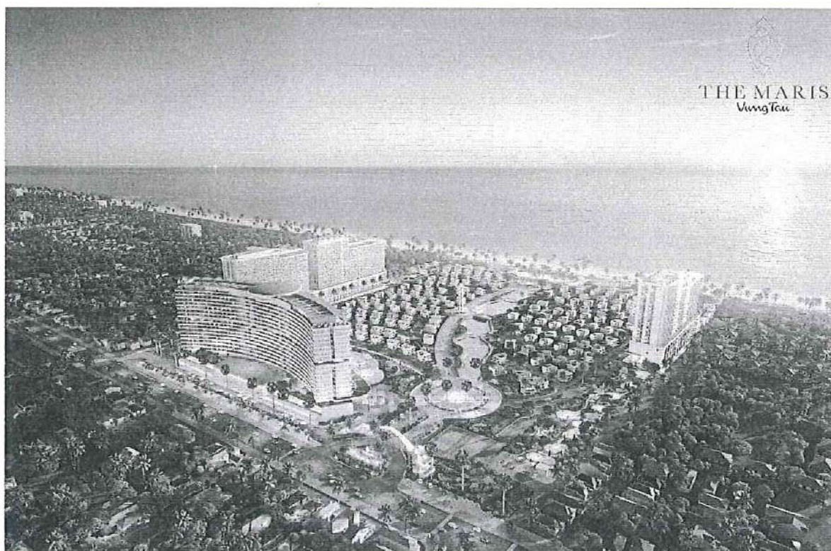
The Maris Vung Tau Project – RYG Porcelain Tiles
